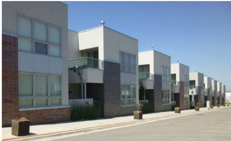
KANSAS CITY, MO - CITY HOMES PROJECT
