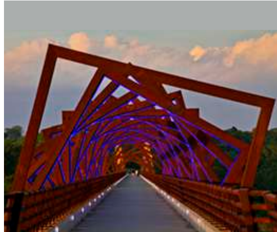
HIGH TRESTLE, CENTRAL IOWA
